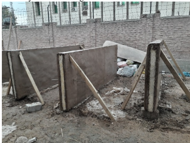
Figure 1: Panels after casting
